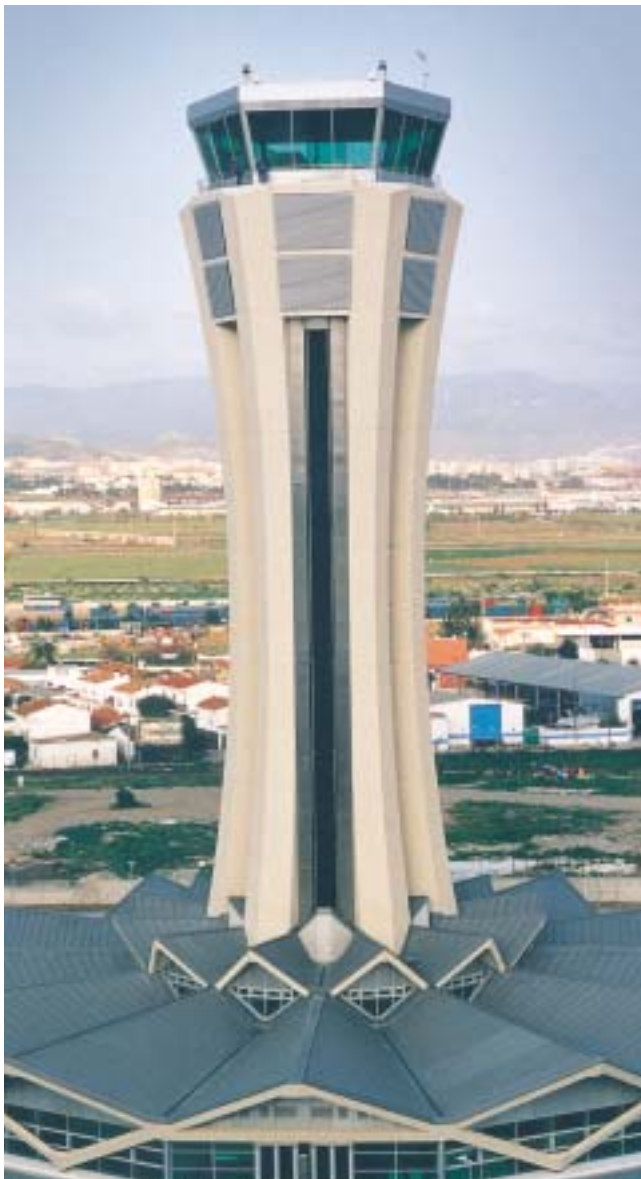
New control tower at the Malaga airport.
