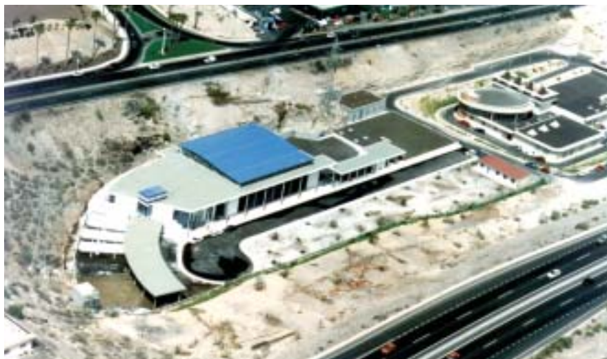
Seawater desalination plant. Adeje-Arona Tenerife.
