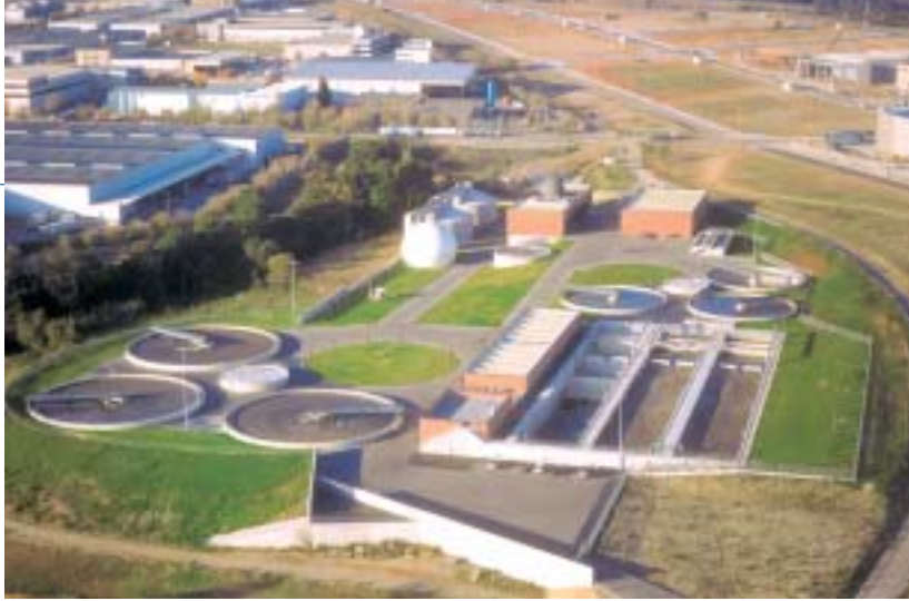
Wastewater treatment plant in Sabadell (Barcelona).
