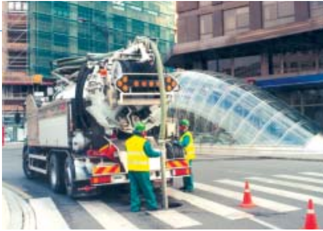
Sewer cleaning, Bilbao.
