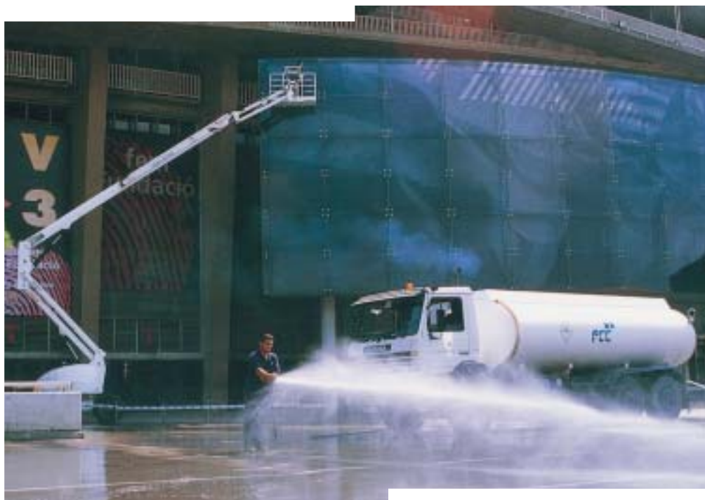
Cleaning of Barcelona Football Club facilities.
