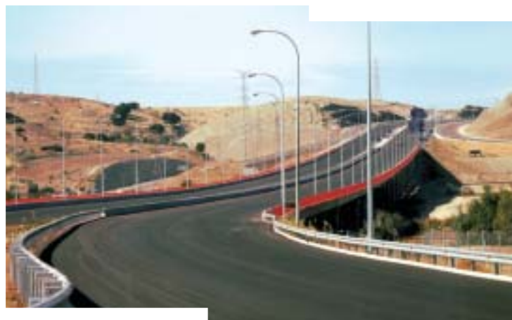
Jarama viaduct on the M-45.
