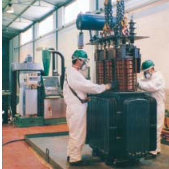
Contaminated transformer maintenance.
