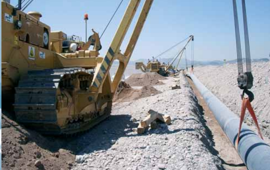
Installation of a primary gas pipeline in Sagunto. Valencia
