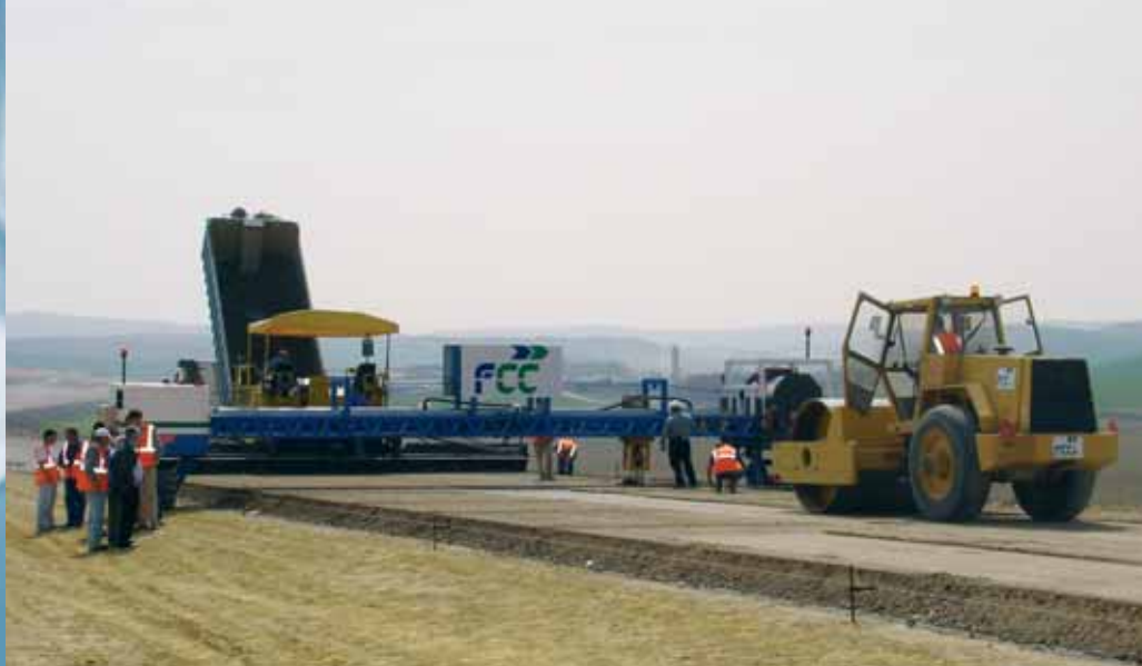
Award promotion of innovation. Design and manufacture of a soil/cement cracking machine
