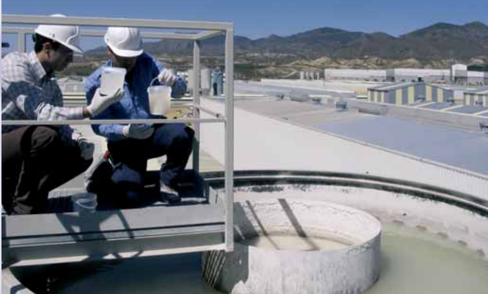
Consentino industrial water treatment plant. Almería
