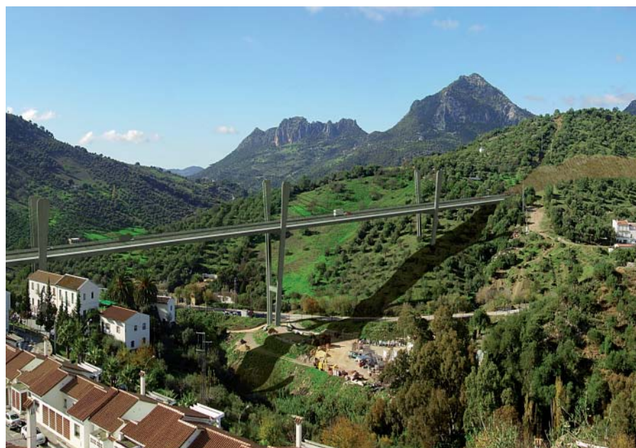
West relief road viaduct in Ubrique. Cádiz
