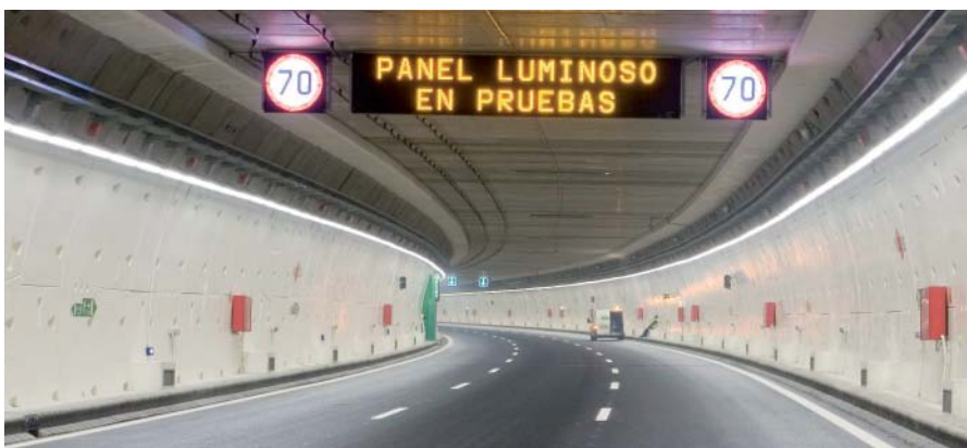
M-30 south bypass tunnel. Madrid
