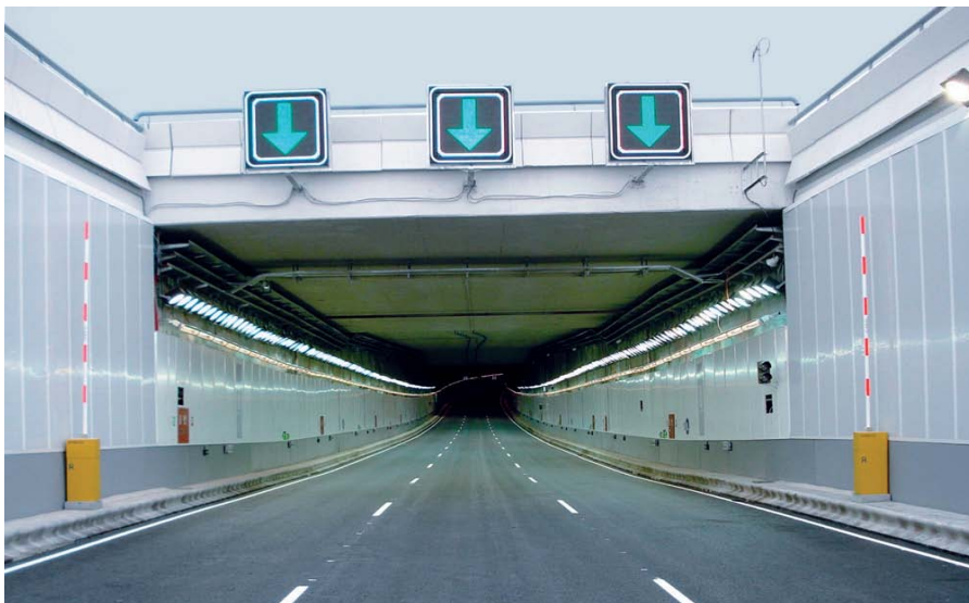
Underground section of the M-30, from Puente de Praga to Nudo Sur
