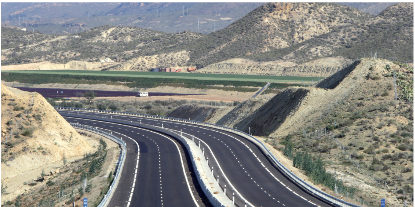
Canero Viaduct. Cantábrico motorway, Querusas - Otur section
